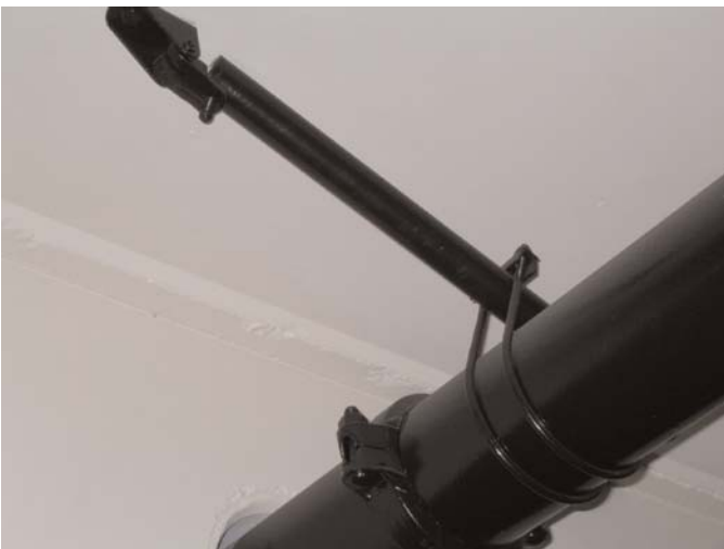
Figure 2 Traditional rigid brace. Photo provided by the author.
